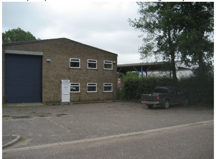
Above a photo prior to the commencement of the existing tenancy
