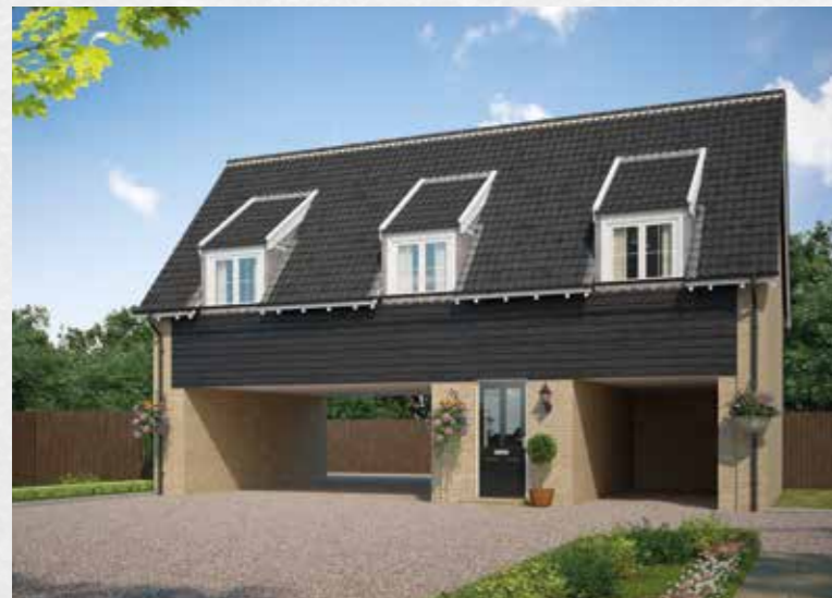
Computer generated image indicative only*. External finishes and appearance likely to vary.
