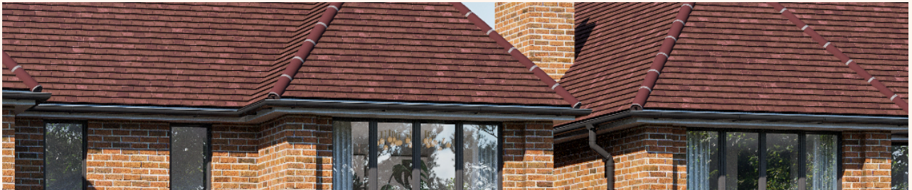
Wienerberger hand-moulded brick, laid with lime mortar beneath a clay peg tile roof
